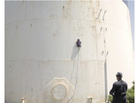
Remote crawler tank shell inspection
